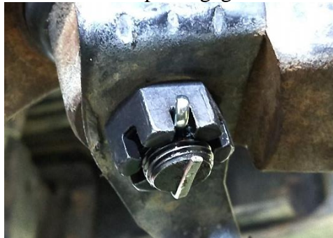
Figure 14. Cotter Pin Installed
