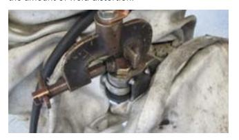
**STEP 7**Weld the back of the bracket to the steering arm.
